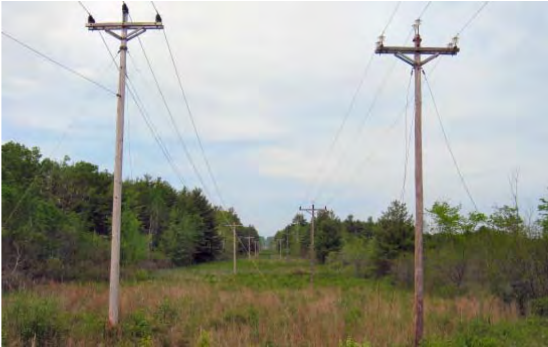
Figure IV-3 – Two 34.5kV sub-transmission lines located on the Unitil system. (Photo by NEI - Unitil System)
