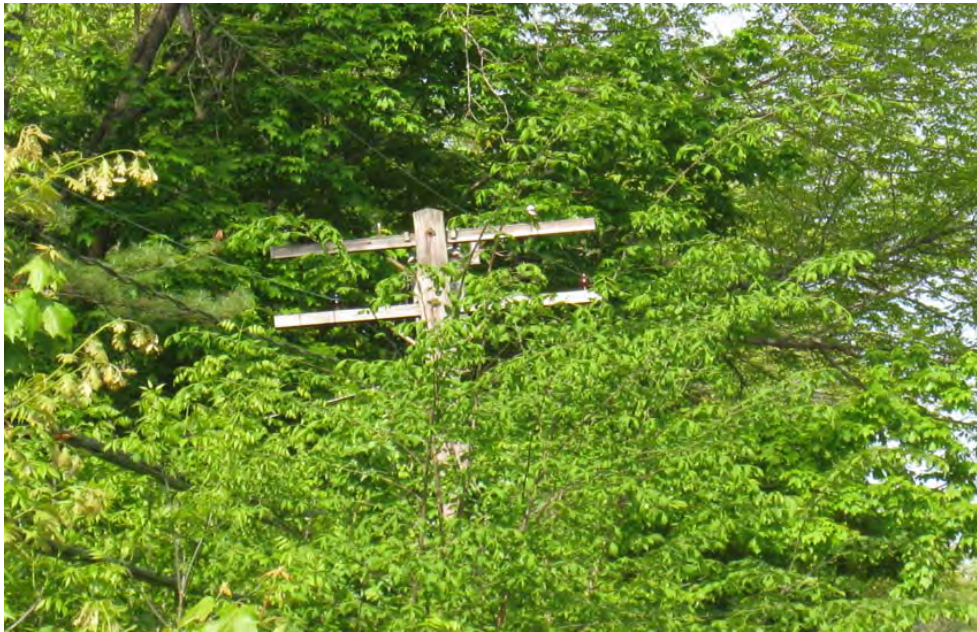
Figure V-14 – NESC Rule 218 violation in Unitil service area. (Photo by NEI)
