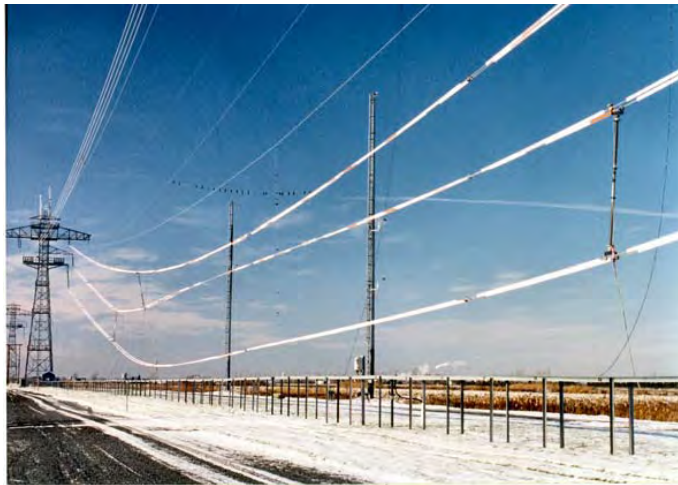
Figure F-9-Excessive sag as a result of galloping. (Photo courtesy of CIGRE)
